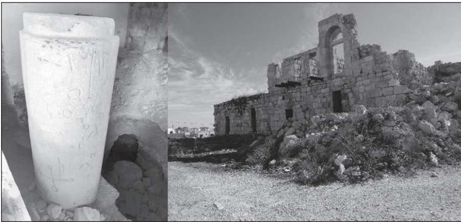
3. Shaft of Roman column used as a foundation or basement of Nabulsi traditional building.
